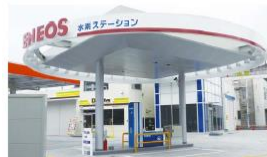
Hydrogen refueling station
